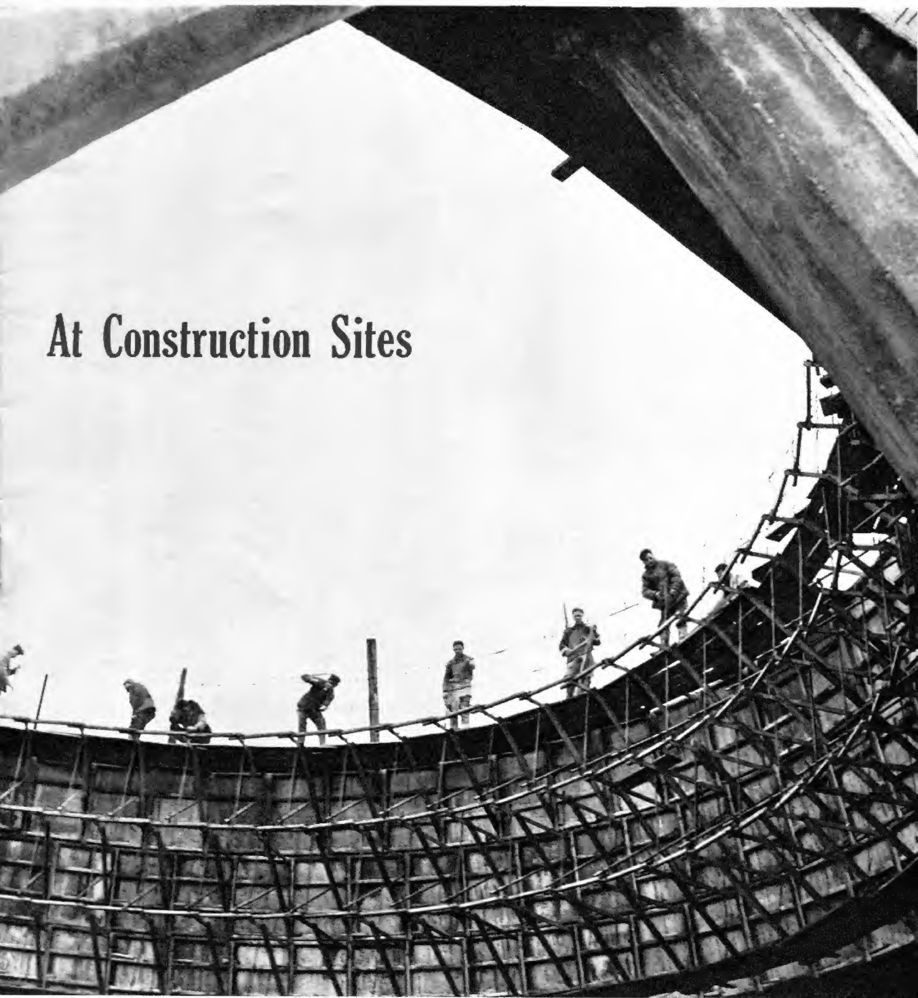
The construction of the tower of the thermoelectric-station in Korea.
